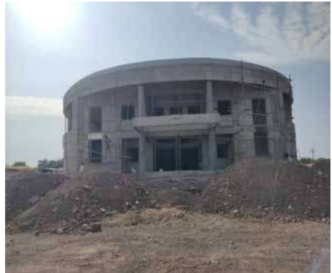
Under-construction building of RC Rajkot
